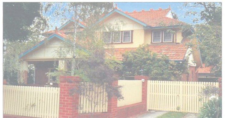
CATEGORY BEST RENOVATION/ADDITION $100,000-$200,000 BUILDER Supa Group Constructions CONTACT Supa Group, 9458 1666 ENTRY Canterbury DESIGNER Supa Group Construction
