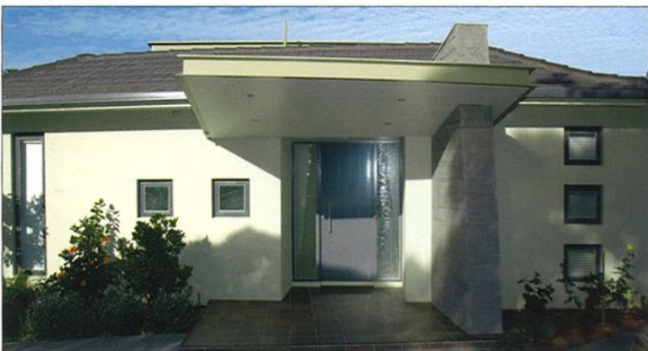
CATEGORY BEST RENOVATION/ADDITION $200,000-$300,000 BUILDER Delroy Constructions CONTACT Joseph Taouk, 9480 1144 ENTRY East Ivanhoe ARCHITECT DeFazio & Co Architects
