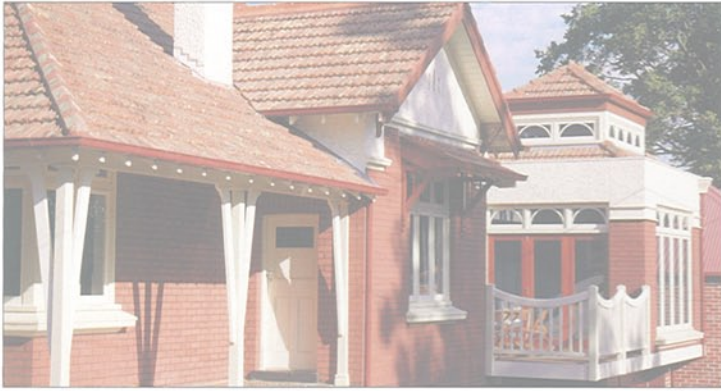
CATEGORY BEST RENOVATION/ADDITION OVER $300,000 BUILDER Hewcon Development Group CONTACT Darryl Hewson, 9499 1262 ENTRY Alphington ARCHITECT Tony Lucas & Associates DESIGNER Interior Rothelwman
